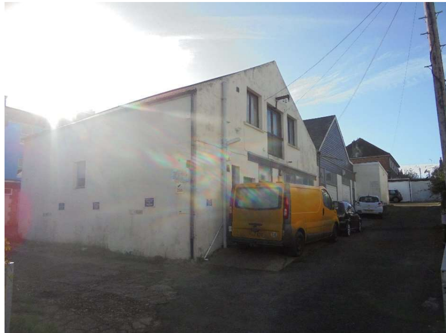
North-east of site
